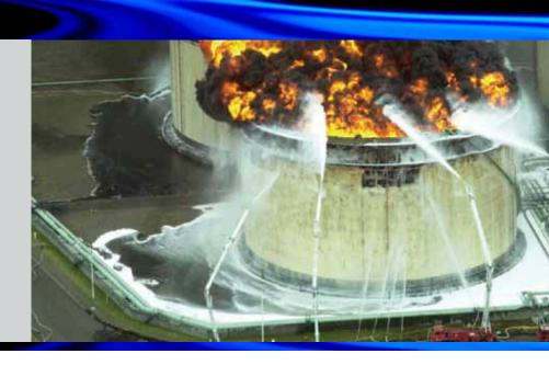
Its unique formulation is based on advanced protein foam technology. The protein base provides a tough cohesive foam blanket with high resistance to heat that quickly smothers, cools, and seals the risk. Fluorochemical surface active agents combined with the protein base increase the fluidity and fuel repellency of the foam.
